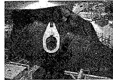
The RSG is lifted onto a purpose-build platform, skidded into the building, and then set into its final position by the containment vessel's internal crane
