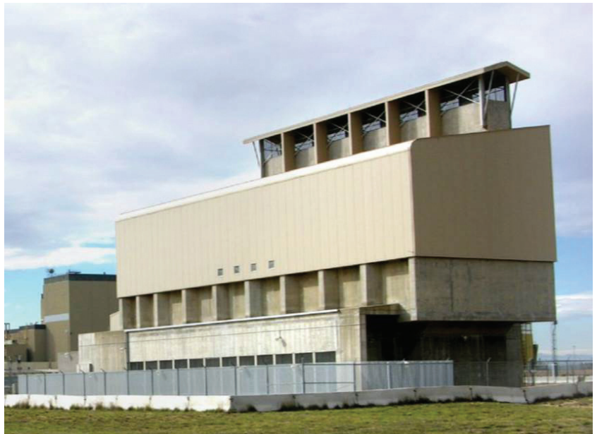
Figure 7-1. Fort St. Vrain independent spent fuel storage installation. The darker building in the background is the decommissioned nuclear power plant, which was converted to a natural gas-fired, electricity-generating station in 1996. (Source: CH2M-WG Idaho 2012).
