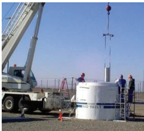
Figure 4-6. Loading TRIGA® spent nuclear fuel into a Rad-Vault for storage.
